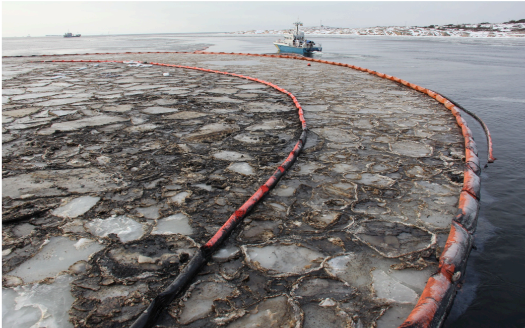
Figure 8: Double Boom Used During the Godafoss Oil-Spill Cleanup, 2011.
