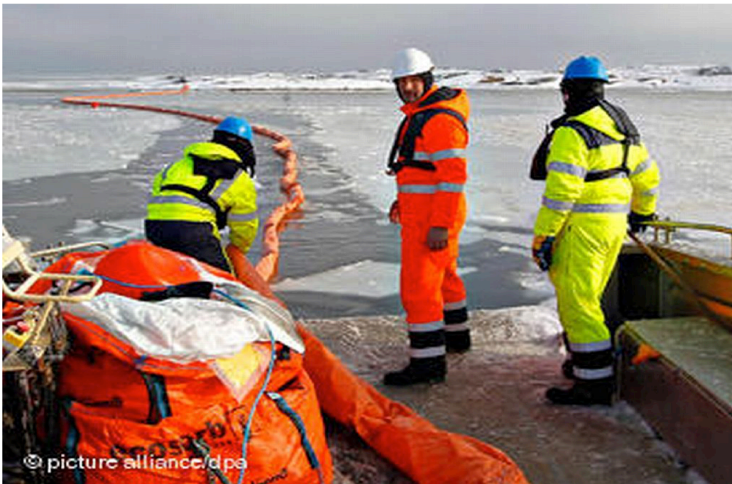
Figure 7: Workers Deploying a Boom during the Godafoss Oil Spill.
