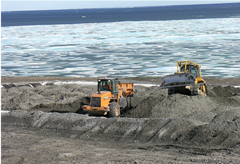
Figure 1: Bioremediation Cleanup of Petroleum-Contaminated Soils on the Coast of Ellesmere Island in the Canadian Arctic, Project Director Dr. Charles Greer (National Research Council Canada, 2016a and b)
