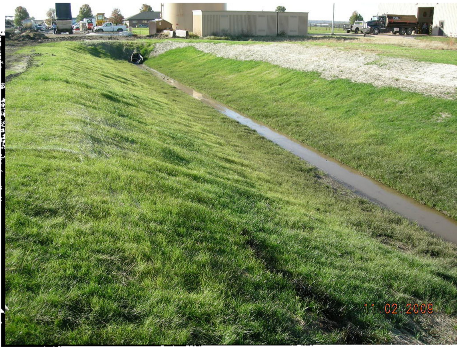
West Detention Pond 11-02-09
