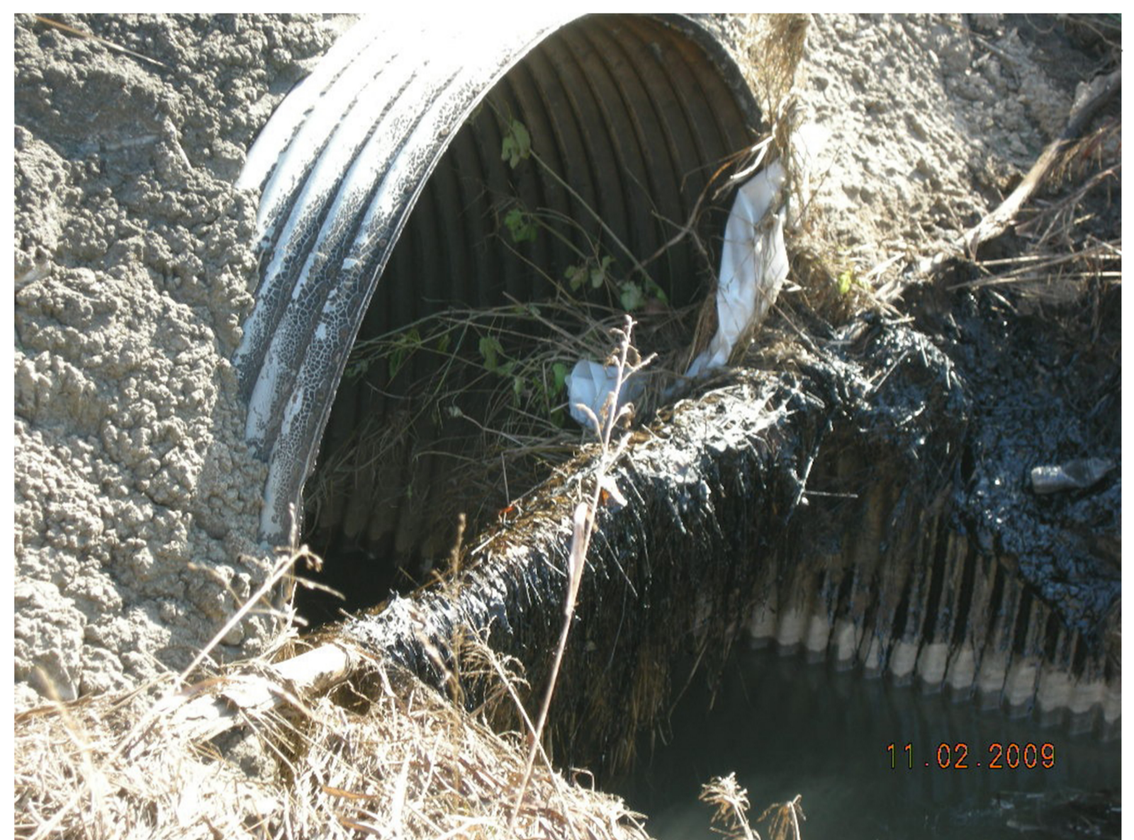
South Ditch 11-02-09 @ South Adams Street
