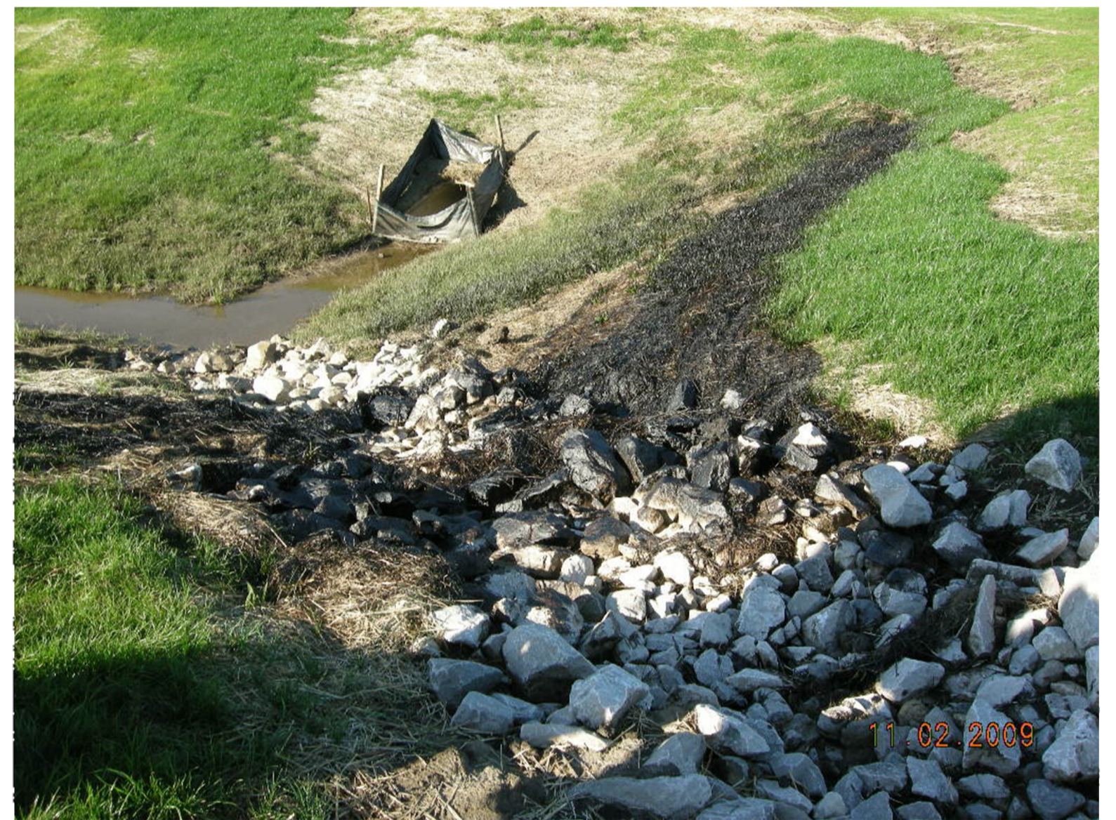
West Detention Pond 11-02-09
