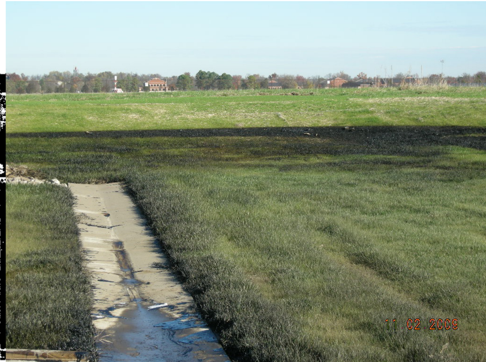
East Detention Pond 11-02-09
