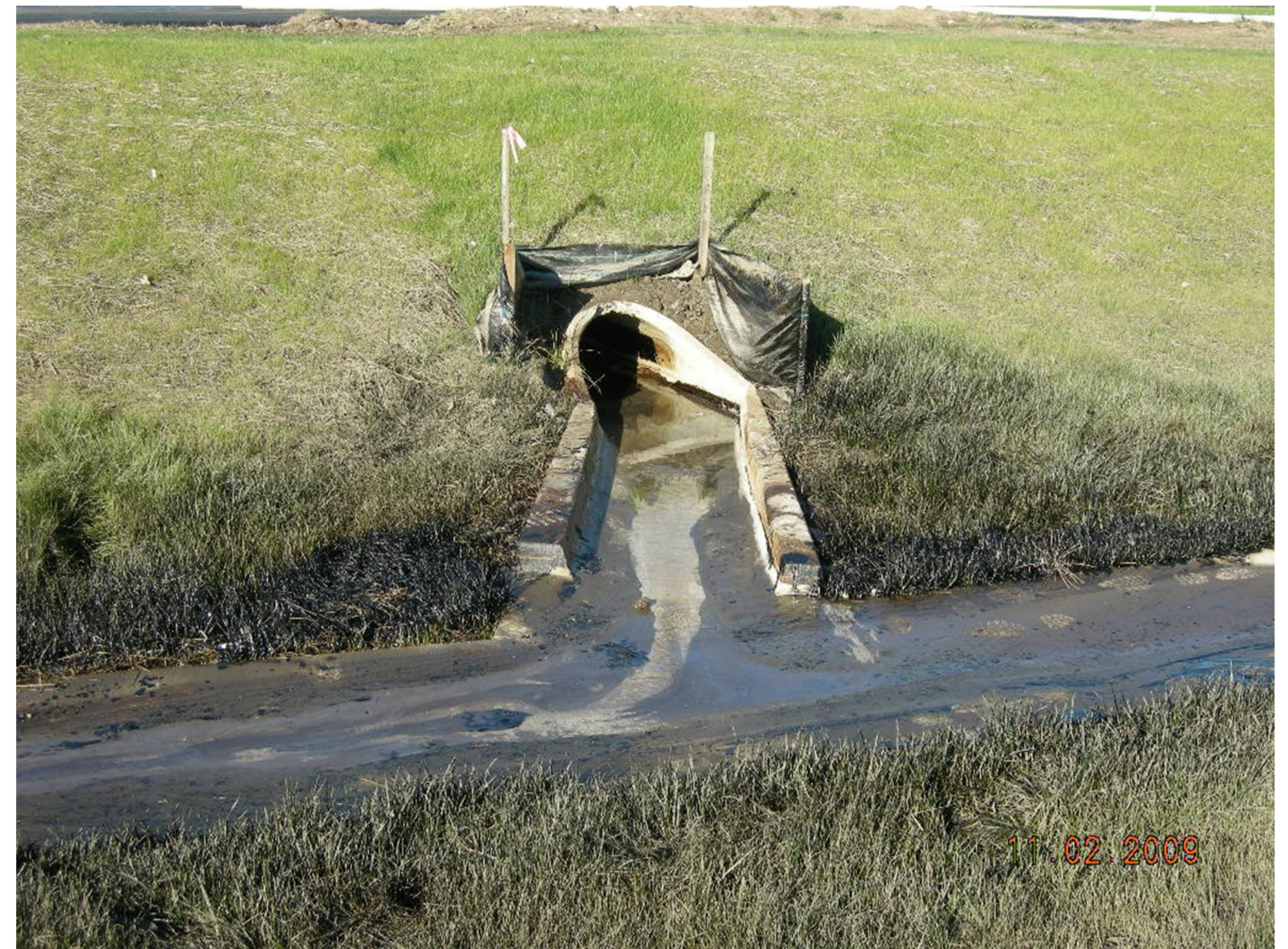
East Detention Pond 11-02-09
