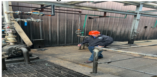
Griffin Pedigo of the OSEI Corporation monitoring the extraction of effluent water with drilling and frac fluids being sent to totes
